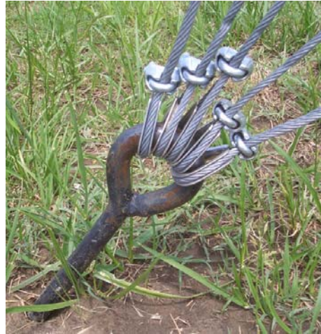
Figure 5, Guy Wire Attachment
